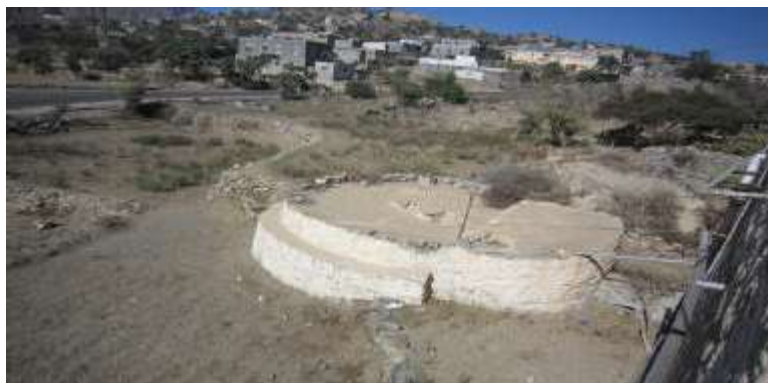
Fig. 3: View of a RTRWHS and pipes (picture taken by Taher)
