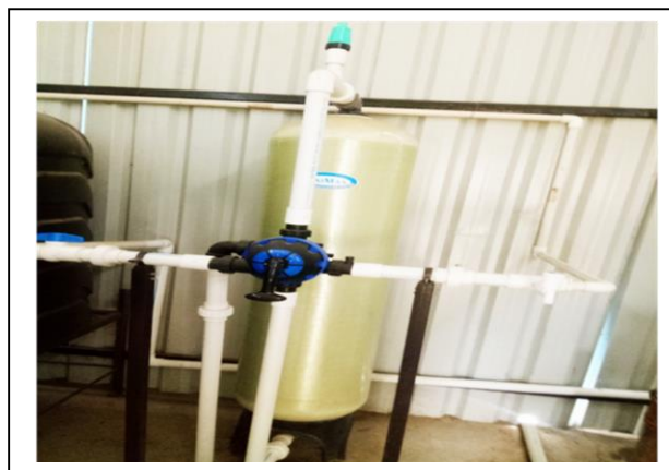
Fig. 3: Dual media filter to remove the Al(OH)_3 flocs from treated water
