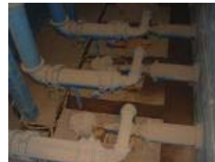
Sand entrance to infrastructures
